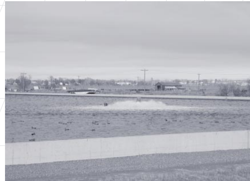
Facultative Lagoon #1 at the Kennewick Wastewater Treatment Plant, Kennewick, WA
