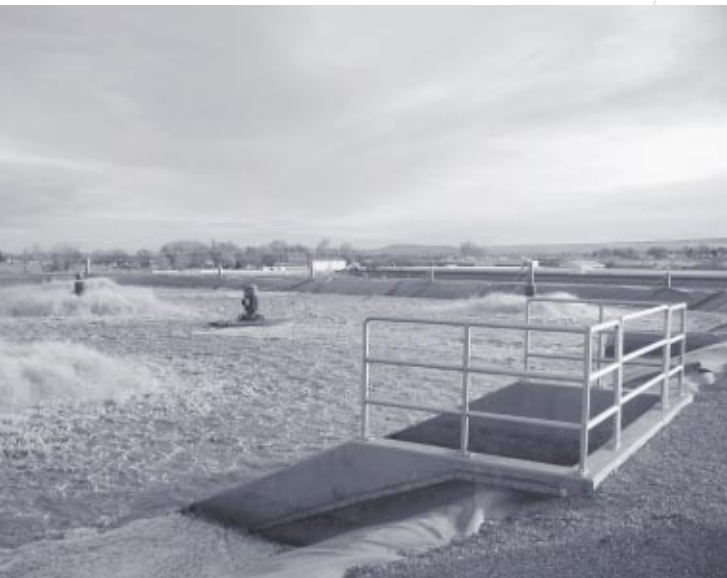
South High Rate Treatment Basin at the Kennewick Wastewater Treatment Plant, Kennewick, WA
