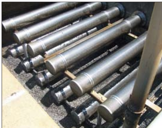
Cylindrical mesh screens keep the media contained to the aeration zone.
