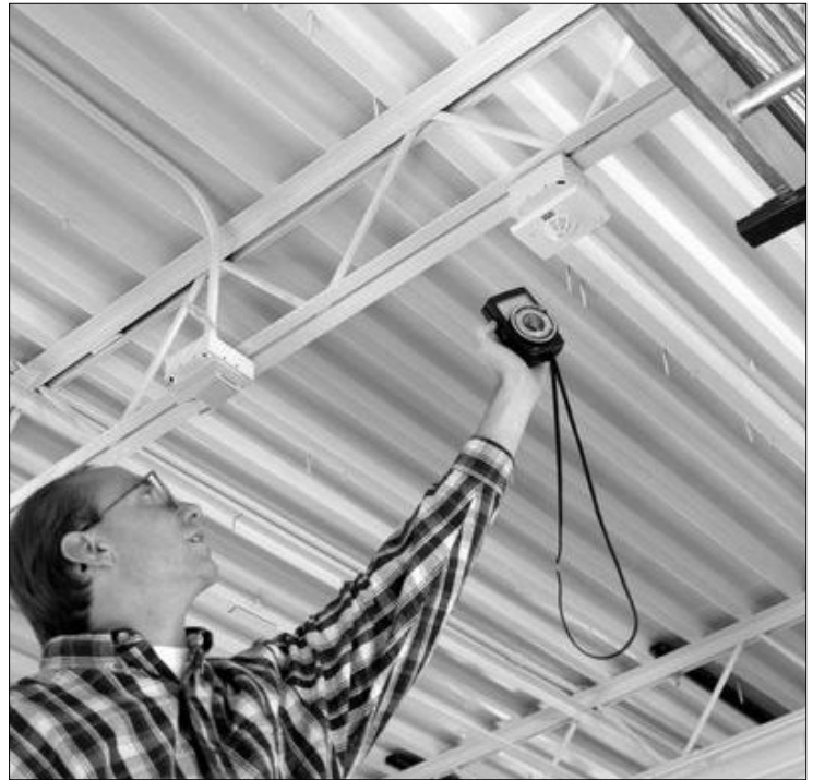
Testing luminance levels is an important part of a retrofitting project.
